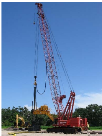
A large diameter auger system will be used during construction activities
